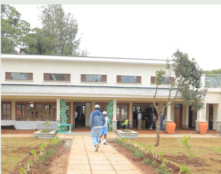
Our new Members' Pavilion is built for generations to come
